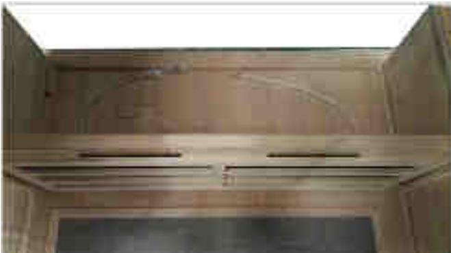
Slide down the bench heater panel by lining up its sides with the vertical guides on left side panel.
